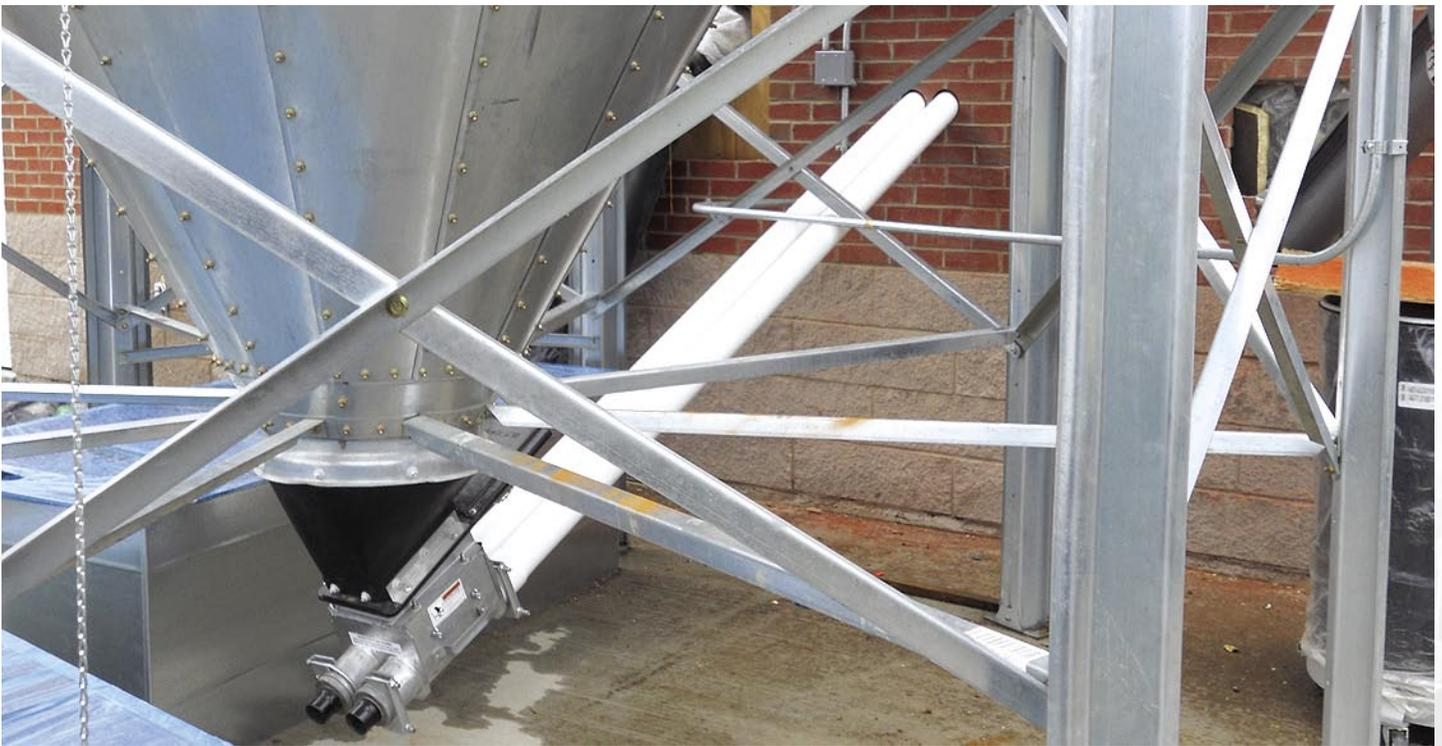
The dual auger system, located at the bottom of the 36 ton silo, automatically delivers pellets to each of the boilers.
