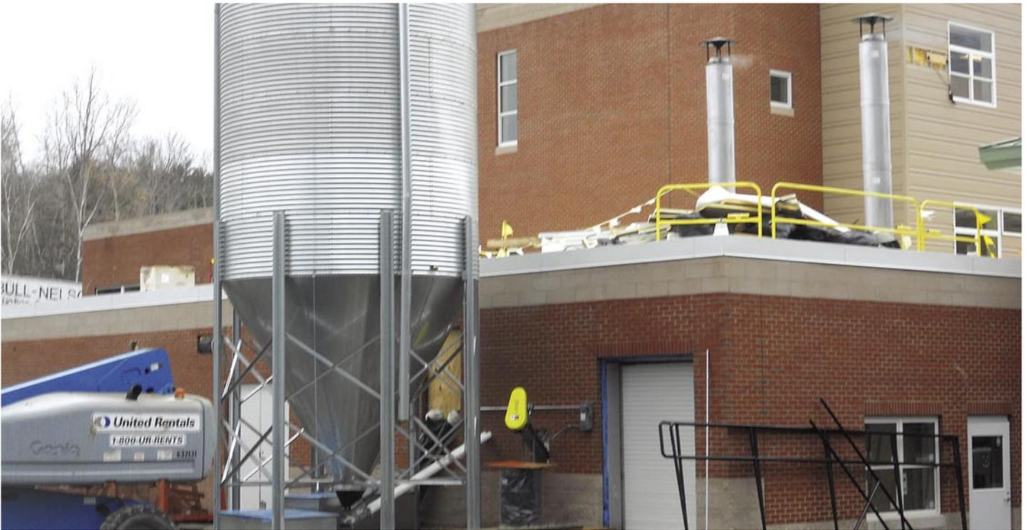
A 36 ton silo located outdoors adjacent to the boiler room stores pellets. The pellets are delivered to each boiler with a dual auger system. During the design process, extensive coordination with the architect and other design team members was required to locate the silo, taking into account proper pellet auger paths, coupled with delivery truck approach and reach.
