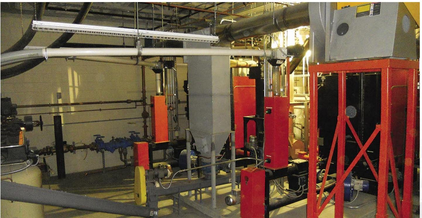
The boilers were equipped with a Multicyclone dust removal system to prevent the emissions of particles greater than 50 microns. The boiler system emissions were modeled as part of EPA compliance requirements.
